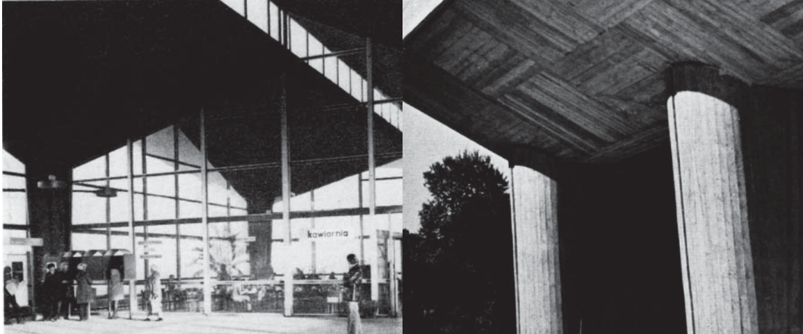
Fig. 1. Interior view of the Katowice main train station, Fig. 2. The pilotis of Le Corbusier's Unite d'Habitation showing the béton brut funnels of its roof structure.
